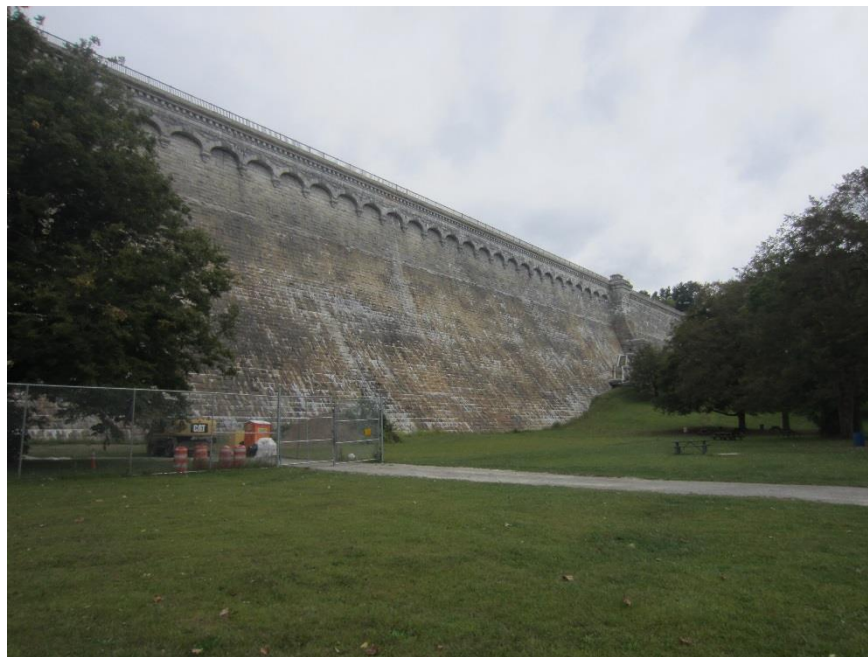
Northernmost injection site near base of New Croton Reservoir Dam
