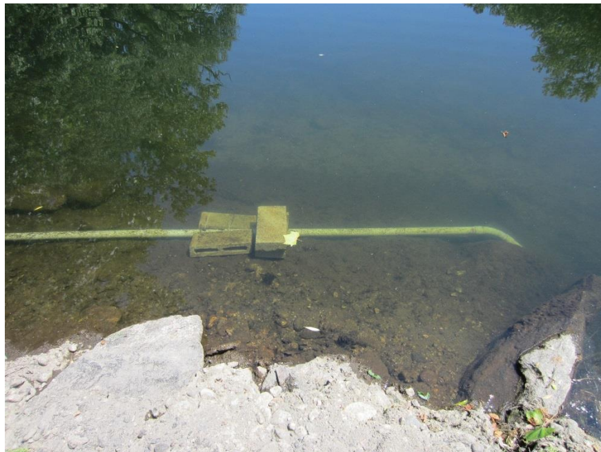
Line from injection unit to release point near Black Rock Dam
